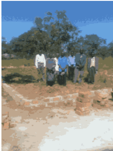
Church building under construction in Chisamba Parish, Zambia
