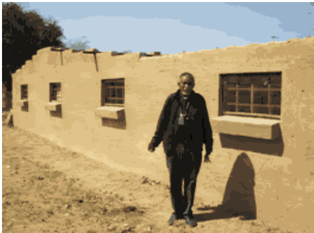
The rebuilt St. Matthew's Parish
